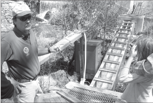
Steve Gephard of the CT DEP at the Mary Steube fishway on the Griswold Preserve. The structure on the left is an eel pass and on the right is a fish ladder.
